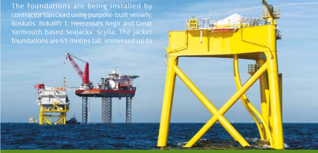
East Anglia ONE jacket foundation, with the substation in the background
