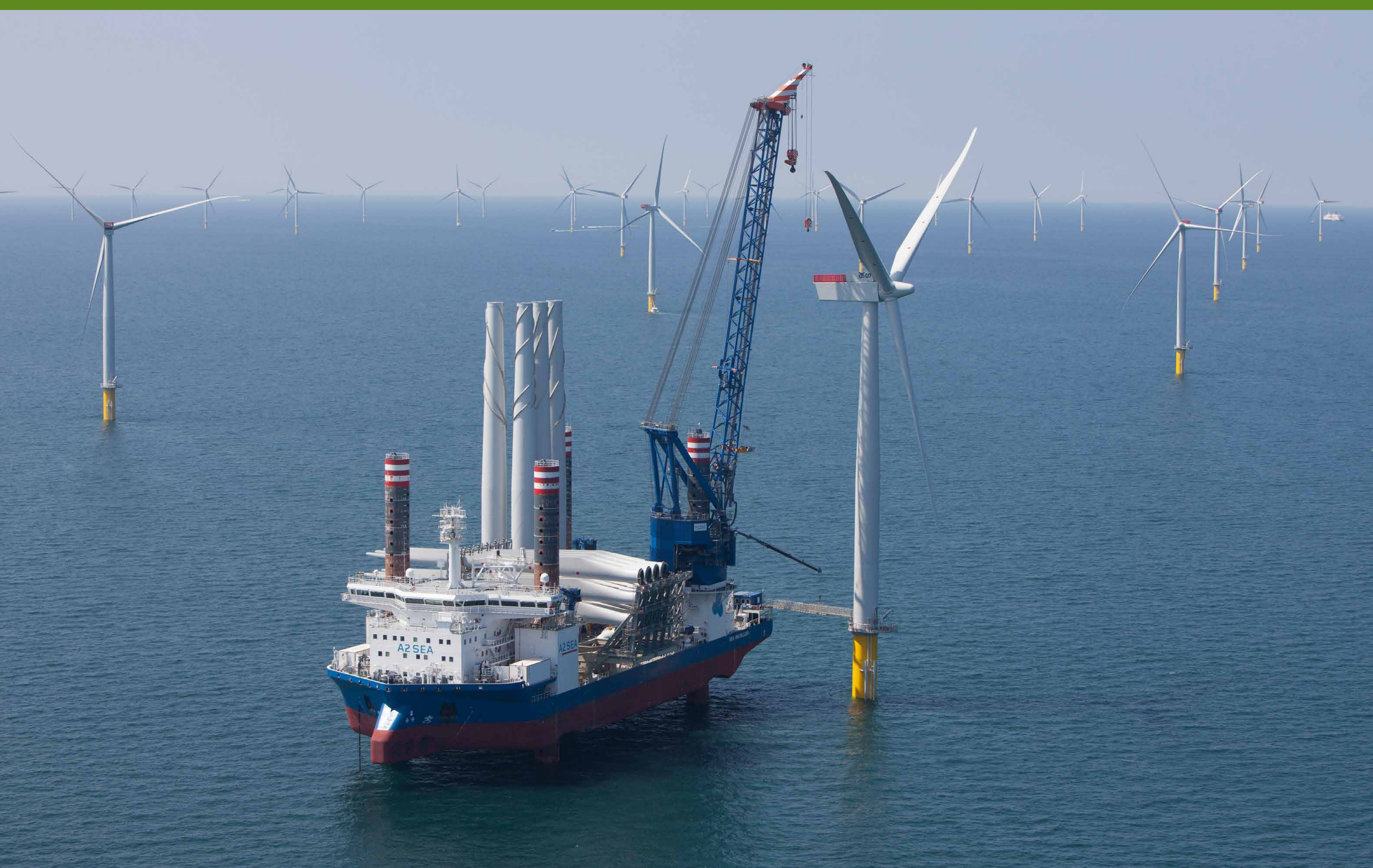
Offshore wind turbine under construction
